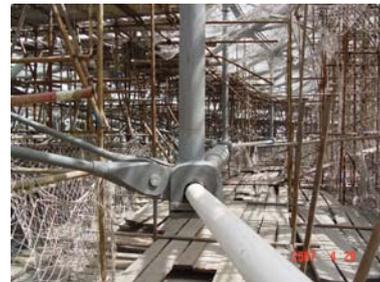
Figure 5. Sliding Cable-strut Joint
