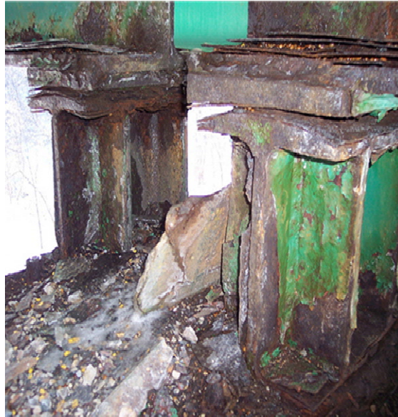
Figure 1. Corrosion Affected Elements of a Steel Bridge
