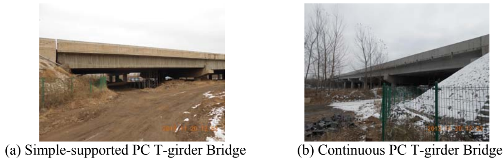
Figure 2. The Two PC T-girder Bridges
