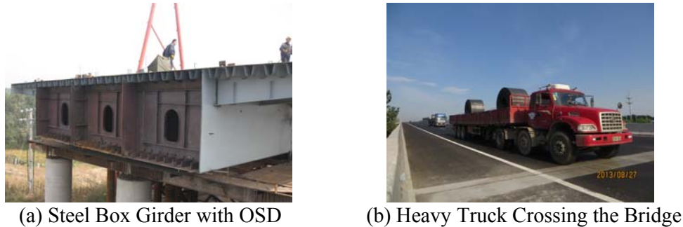
Figure 1. Houdingxiang No.1 Bridge with OSD
