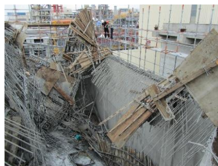
Fig. 1 Scene of the collapse of falsework in construction of an iron & steel company in Central Taiwan
