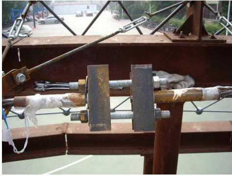
(a) Before pre-stressing construction
