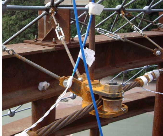
Figure 9. Photo of the Rolling Cable-strut Joint
