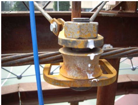
(a) Before pre-stressing construction
