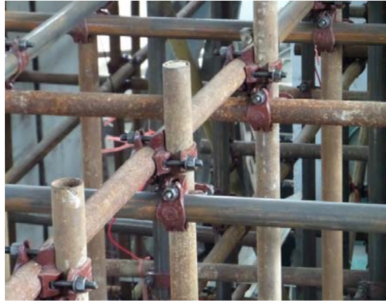
Figure 11. Connection of Horizontal and Vertical Members in Coupler-type Scaffold Structure
