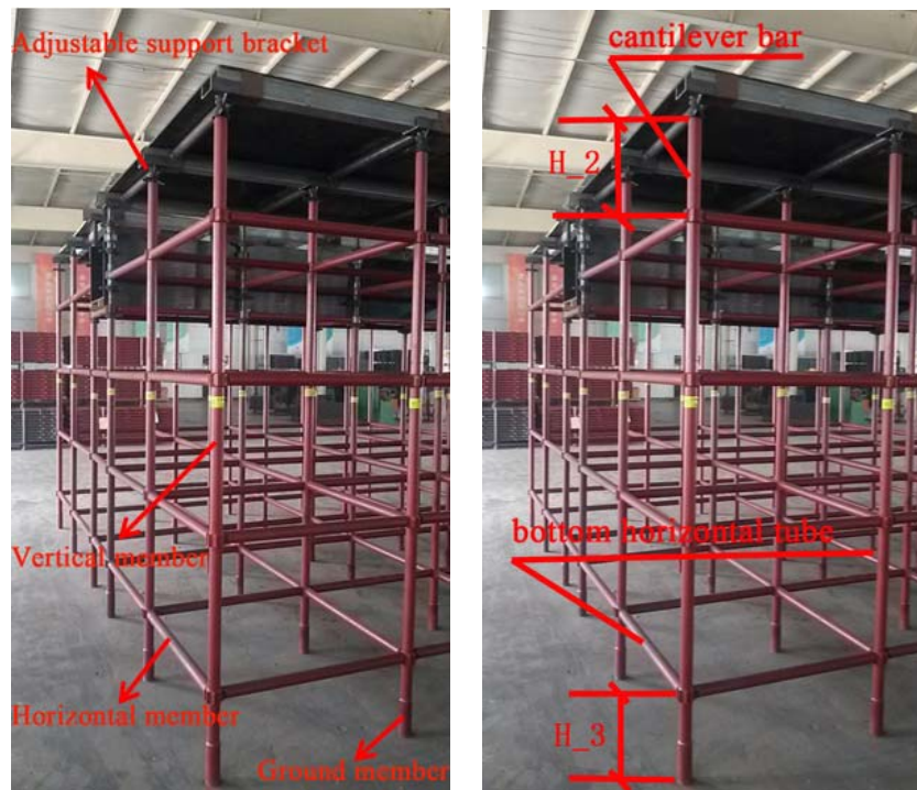
Figure 2. Structure of Mortise-tenon Steel-tube Scaffold
