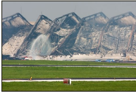
Figure 1. Collapse of the Aircraft Warehouse of Brussels International Airport after Fire
