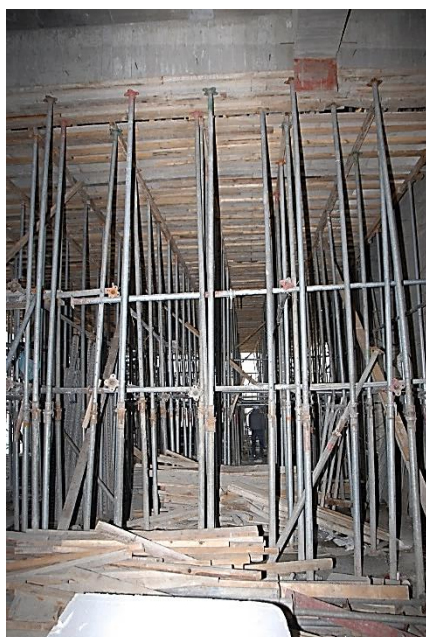
Fig. 1 A single-story temporary support on a construction site in Taiwan
