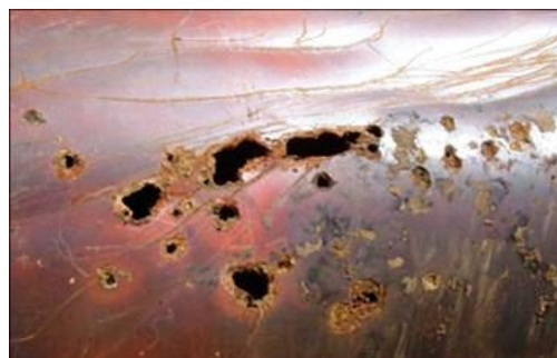
Fig. 1 Metal pitting corrosion
