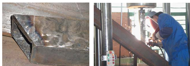
Figure 1. Fabrication of A Square Tubular Y-joint
