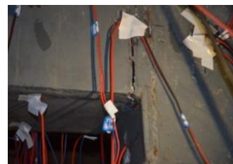
Fig. 10 Final failure mode of JD-2 (mode II)
