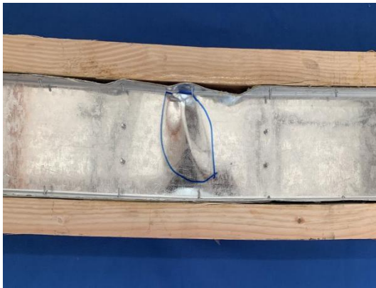
(c) Buckling of the section web observed at the L-6 beam
