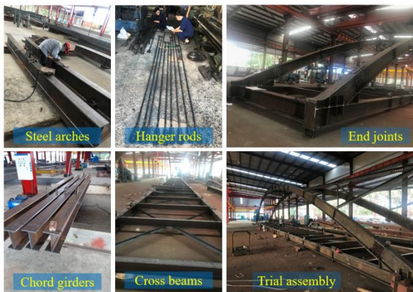
Fig. 22 Fabrication and trial assembly of the steel structures at the factory
