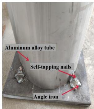
(a) Connection between aluminum alloy and end plate
