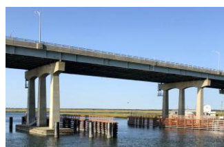
(a) Steel girders used in marine structures
