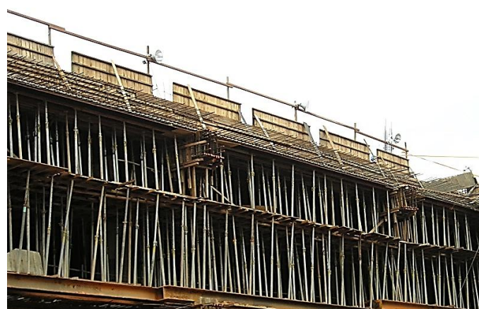
Fig. 2 A double-story temporary support on a construction site in Taiwan
