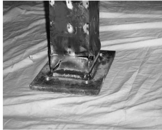
Figure 8. Fracture of member S-5-0
