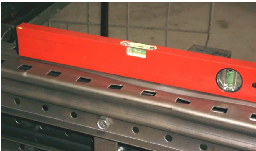
Figure 10. Local Buckling of Column Web in Compression Zone
