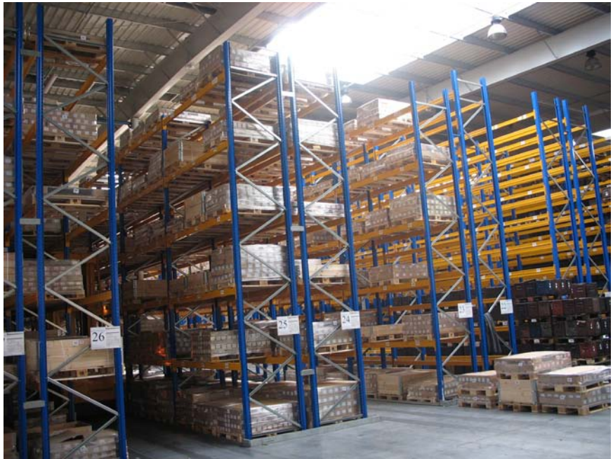
Figure 1. Typical Pallet Racks Configuration
