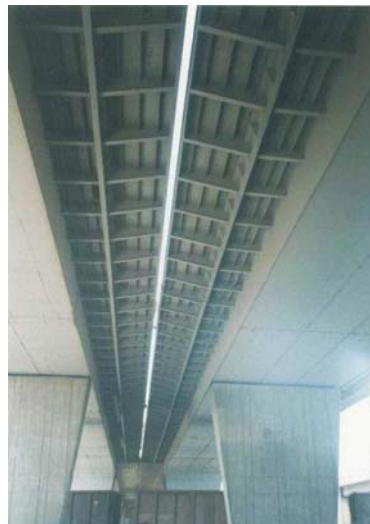
Figure 18. A View from Beneath the Orthotropic Bridge
