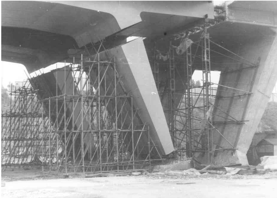
Figure 11. Assembling of the Steel “V”- Supports
