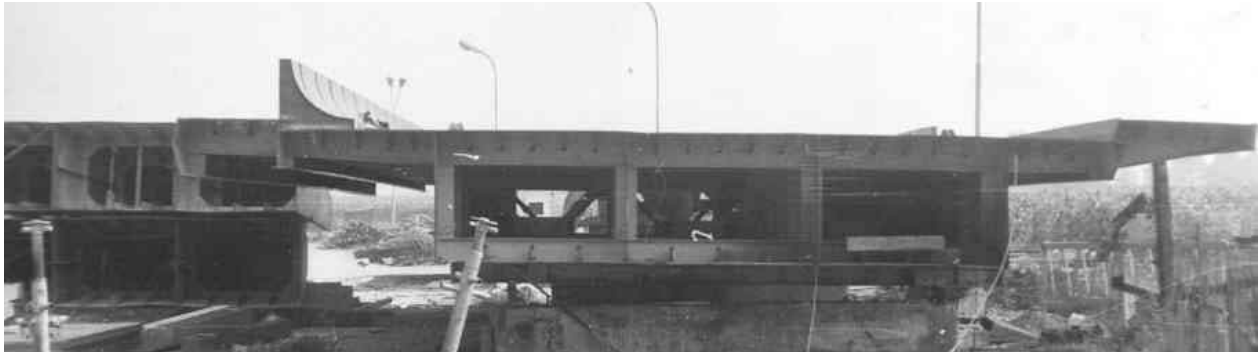
Figure 5. Triple-Box Section of the Bridge Deck
