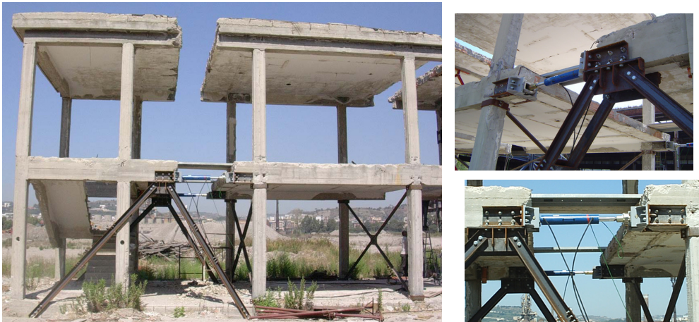
Figure 10. Pushover Test on the Module under Study
