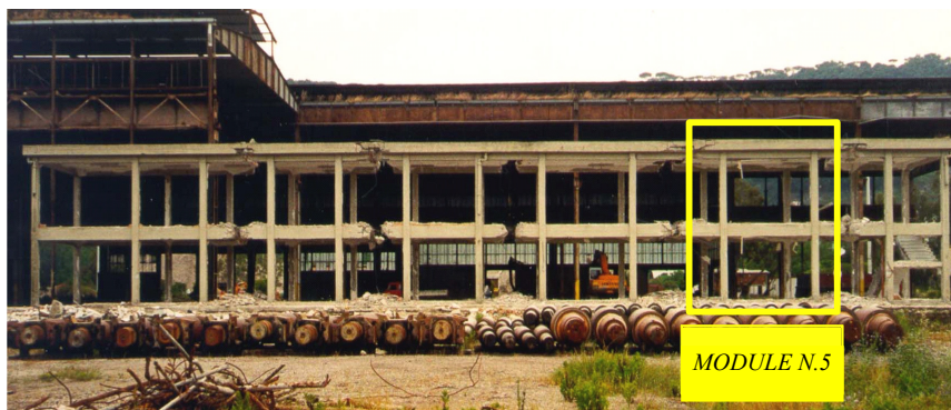
Figure 5. The Division in Sub-structures (Modules)
