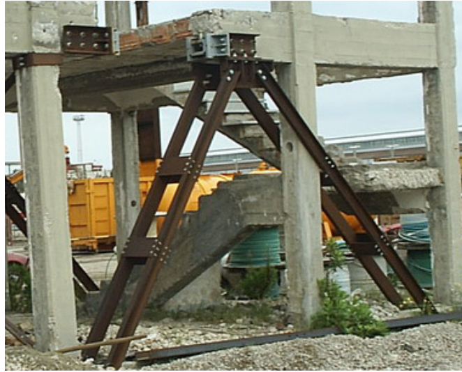
Figure 23. The Retaining Steel Structure
