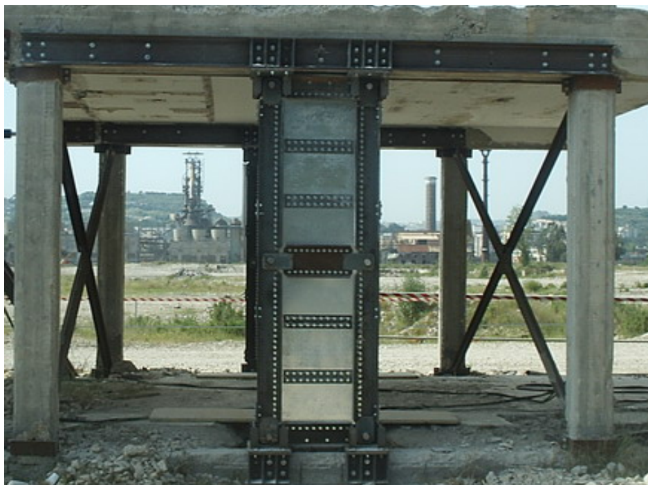
Figure 22. Global View of the Retrofitted Structure
