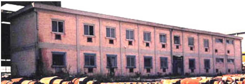
Figure 4. The Original Building
