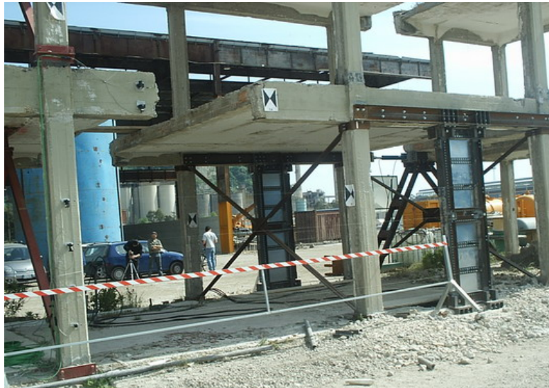
Figure 25. Global View of the Measurement Devices Applied on the Upgraded Structure
