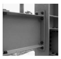
Figure 1. Bolted Extended End-Plate Connection
