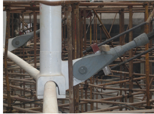
Figure 8. Sliding Cable-strut Joint
