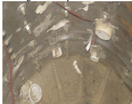
(a) Internal Wall
